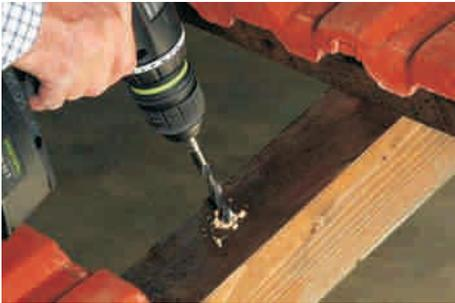
3: Drill rafters  $\varnothing$  8mm
