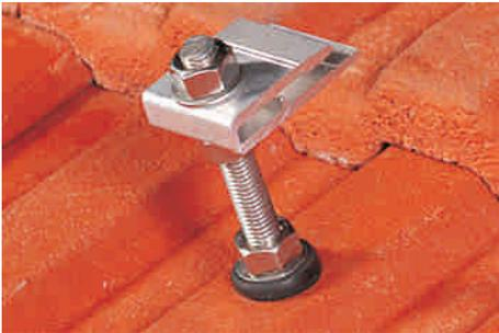
6: Set the clamping pieces to a common height and secure them (distance from top edge of the brick to bottom edge of the clamping piece approx. 20-30mm)
