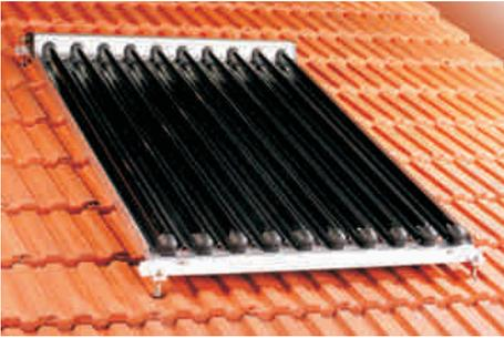
8: Insert the collectors and attach them to the support rails with screws.
